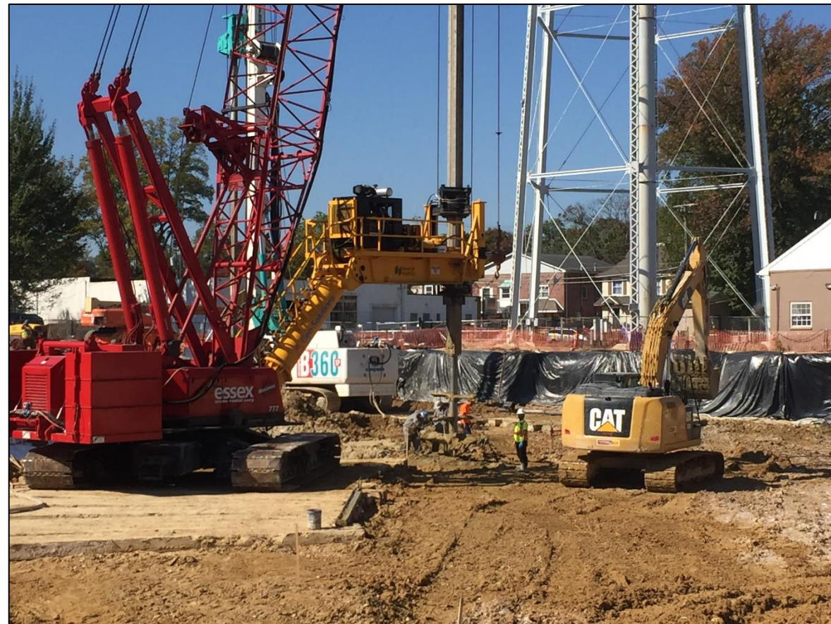
HAMMONTON: TREATMENT VIA IN-SITU SOIL SOLIDIFICATION / STABILIZATION (ISS)
