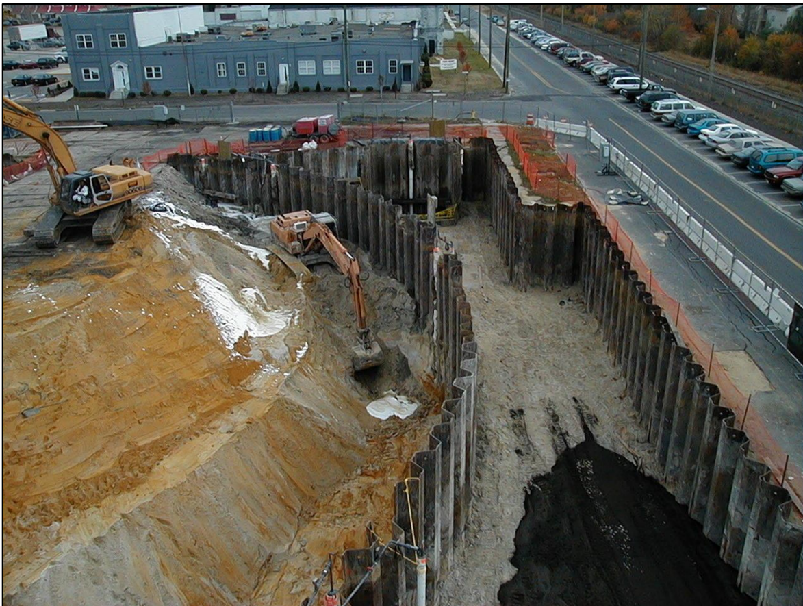
EGG HARBOR CITY: REMOVAL VIA EXCAVATION AND THERMAL DESORPTION TREATMENT
